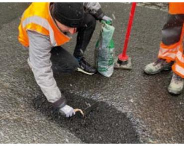
Under strict quality assurance control, important production properties such as temperature, binder ratios and the granulometry etc. are ensured. This control ultimately results in this unique, long-lasting, cold-processable hot asphalt product that can be stored for up to 36 months.
